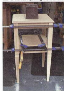
27 Fit the lower shelf in two halves rejoining them in situ.
